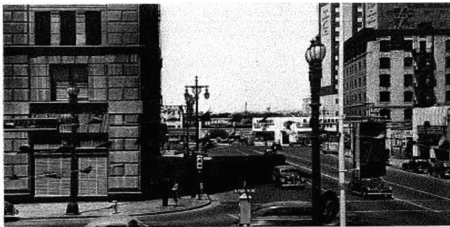
Olympic Boulevard and Flower Street, 1941, the Widening Job Completed
