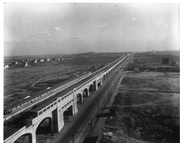
Figure 1: Elevated IRT 7 Fortieth Street station under construction, Queens, 1917. Source: New York City Metropolitan Transit Authority.
