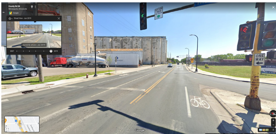
(b) The same grain silos, viewed from 75 meters distance.
