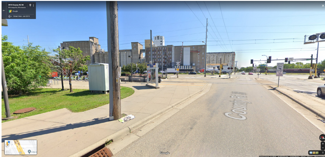
(a) Grain silos on 38th Street and Hiawatha viewed from 150 meters distance.
